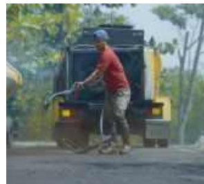
Gambar 5. Penerapan Tack Coat
