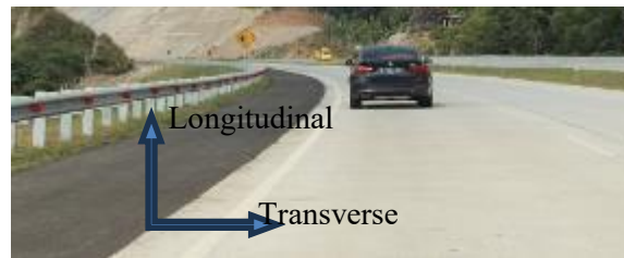
Figure 2. Longitudinally Laid Composite Pavement on Cipali Highway
