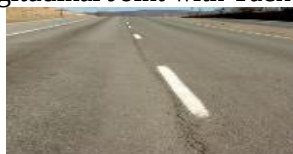
Figure 11. Example of Longitudinal Joint Failure
