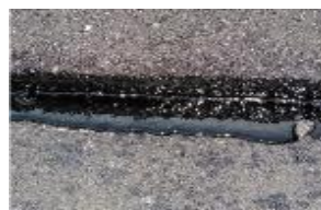
Figure 10. Longitudinal Joint with Tack Coat in Minnesota
