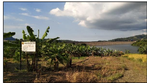
Figure 6. Farm Corp At The Dam Hazard Zone, 2019.
