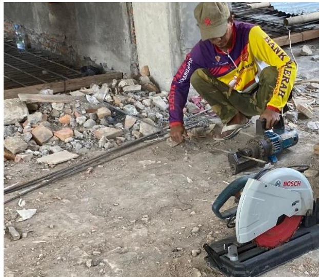
Figure 4. Cutting Reinforcing Steel
