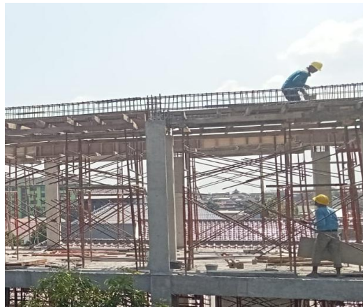
Figure 7. Tying Reinforcement Connections with Wire Hooks
