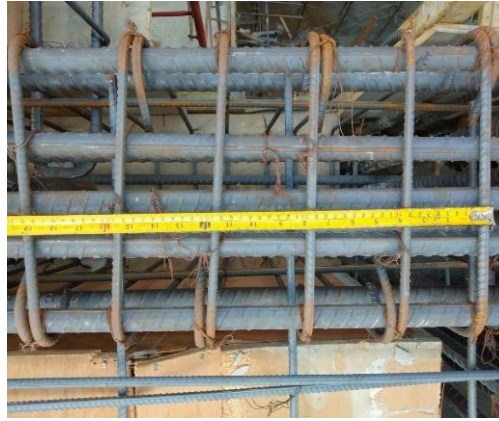
Figure 6. Measurement of Distance between Rebar
