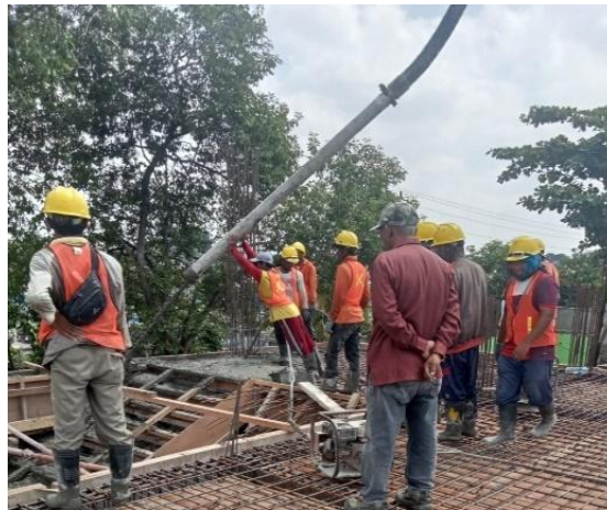
Figure 13. Pouring fresh concrete using a pump truck
