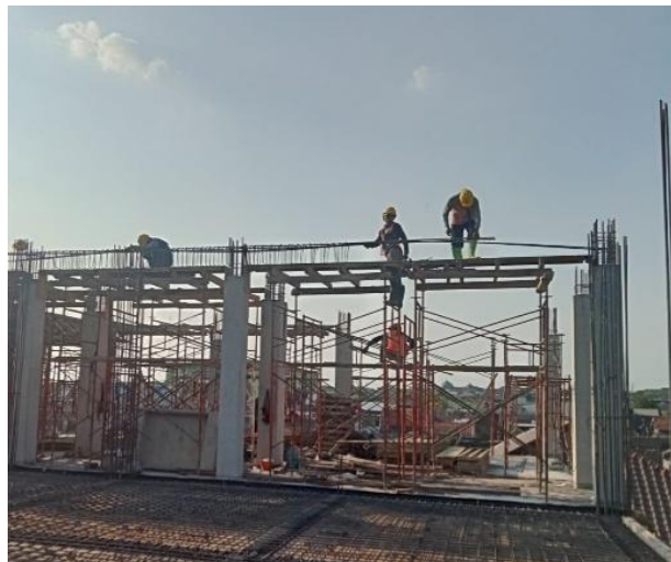
Figure 5. Installation of Main Reinforcement
