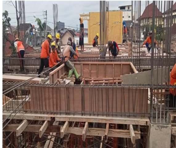
Figure 9. Installing formwork on scaffolding
