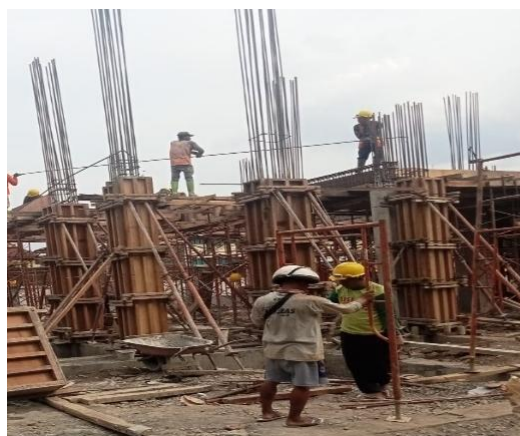
Figure 8. Installation of scaffolding on formwork
