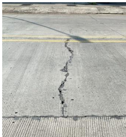
Figure 4. Linear Cracking Damage
