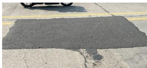
Figure 5. Patching Damage
